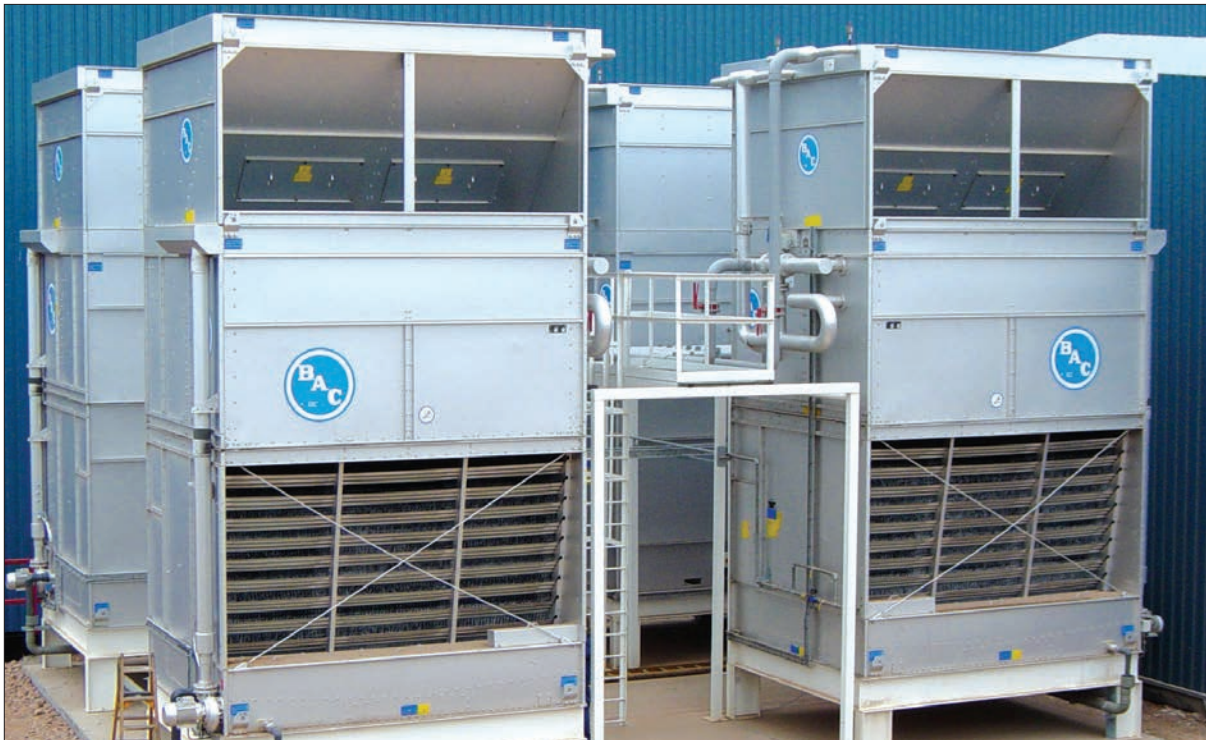
Multi-cell HXV Installation
