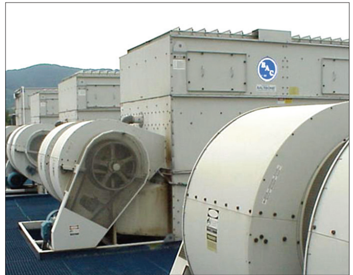
Multi-cell VFL Installation
